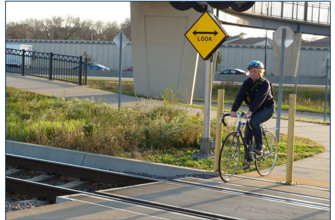
Signs and railroad crossing lights guard trail crossing of Hiawatha light rail corridor; Minneapolis, Minnesota – Stuart Macdonald, americantrails.org
